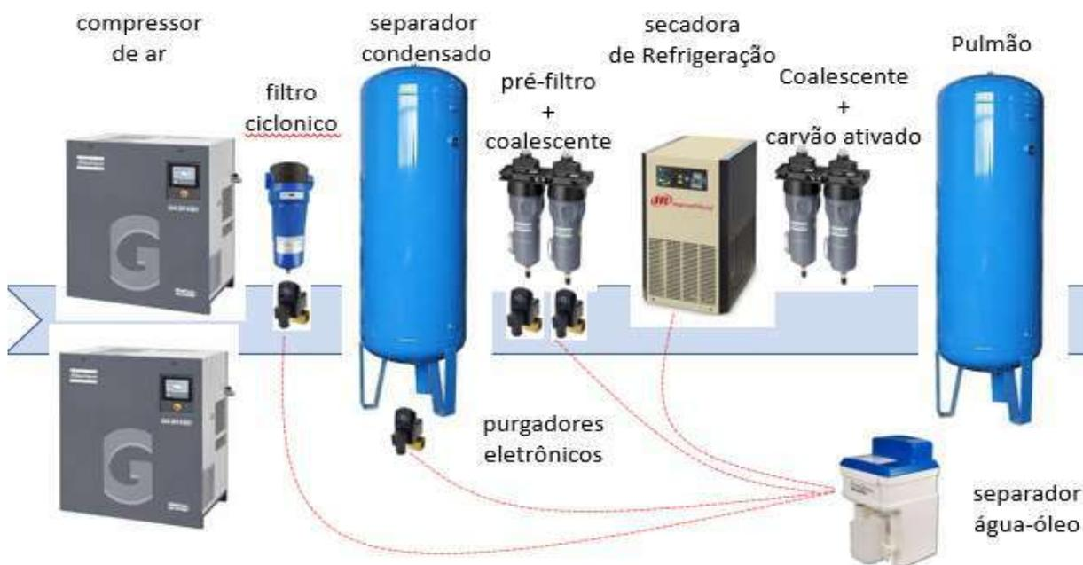
**FOTO ILUSTRATIVA DO SISTEMA DE AR COMPRIMIDO MEDICINAL**
